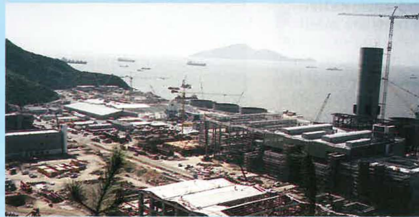
Progress at Black Point. 爛角咀發電廠
